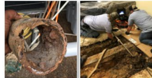
JSC Potable Water
